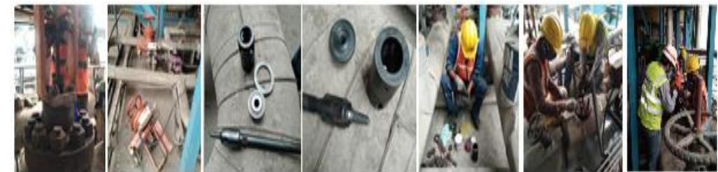
Control Valve Dismantling, Gasket Replacement, stem, seat, cage, aping, blue matching & calibration
